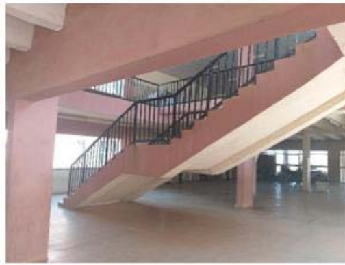
Plate 2: Public staircase within the hospital. August 2018
