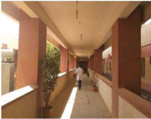
Plate 1: Corridor as a physical feature within the hospital. August 2018
